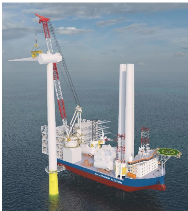
Figure 2: NG-20000X installing a WTG.
